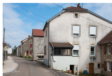
Maison, Grande rue. Phot. Jérôme Mongreville IVR43_20187000093NUC4A
