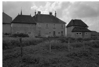
Façade postérieure. Phot. Gilbert Poinot IVR43_19752500814Z
