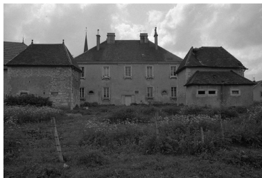
Façade postérieure. Phot. Gilbert Poinot IVR43_19752500815Z
