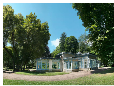
Façade est, vue en 2008. Phot. Pierre-Marie Barbe-Richaud IVR26_20085800007NUC2AQ
