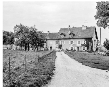
Habitation principale. Phot. Dominique Dominguez IVR43_19807000273X
