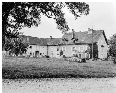
Habitation principale. Phot. Dominique Dominguez IVR43_19807000274X
