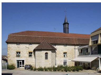
Façade postérieure. Phot. Michel Thierry IVR26_20047101074NUC2A
