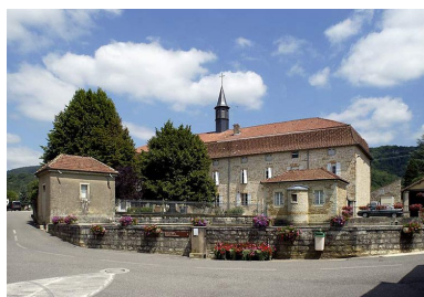
Façade antérieure. Phot. Michel Thierry IVR26_20047101093NUC2A
