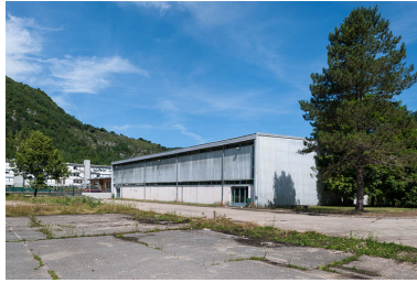
Gymnase. Phot. Jérôme Mongreville IVR43_20143900448NUC4A
