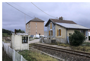
Façades sud et est. Phot. Yves Sancey IVR43_20043900272ZA
