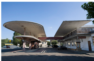
Gare et station bus. Phot. Yves Sancey IVR43_20067000891NUCA
