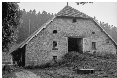
Façade postérieure. Phot. Gilbert Poinot IVR43_19752501324Z
