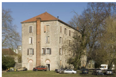
Pignon sud. Phot. Jérôme Mongreville IVR43_20097000197NUC2A
