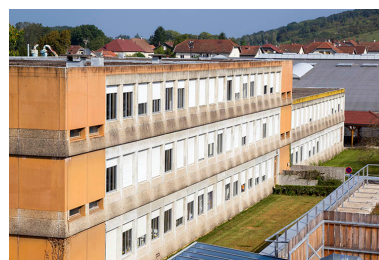
Externat : façade est. Phot. Sonia Dourlot IVR43_20143900657NUC2A
