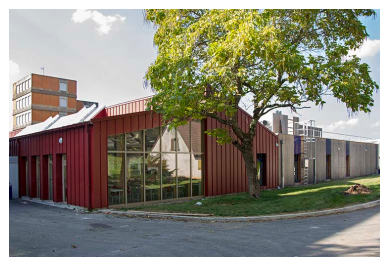
Restauration : façades. Phot. Sonia Dourlot IVR43_20143900662NUC2A
