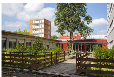
Restauration : patio. Phot. Sonia Dourlot IVR43_20143900678NUC2A
