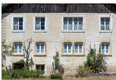
Façade antérieure. Phot. Sonia Dourlot IVR43_20162500860NUC4A
