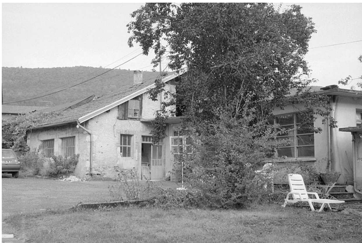
Ateliers de fabrication (E, F).
