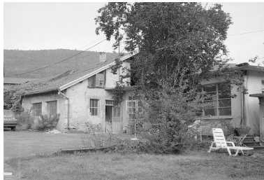
Ateliers de fabrication (E, F). Phot. Laurent Poupard IVR43_19913901090Z
