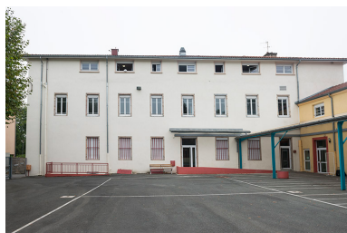
Internat : façade postérieure. Phot. Mary Ruffinoni IVR43_20143900777NUC4A
