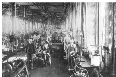
Atelier de construction. Phot. Jérôme Mongreville IVR43_20029000012X
