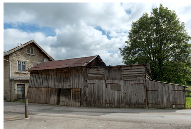
Ateliers de menuiserie. Phot. Sonia Dourlot IVR43_20162500639NUC4A
