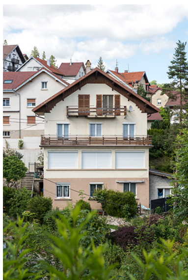
Façade postérieure. Phot. Sonia Dourlot IVR43_20162500888NUC4A
