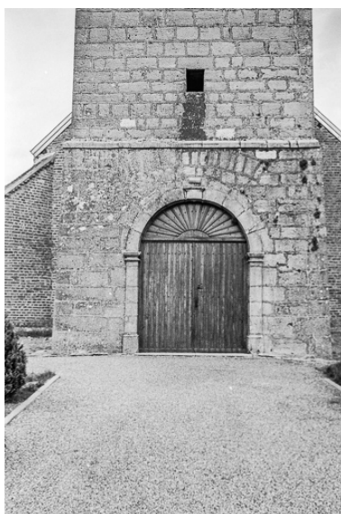
Portail. Phot. Guy Forestier IVR43_19753900145Z
