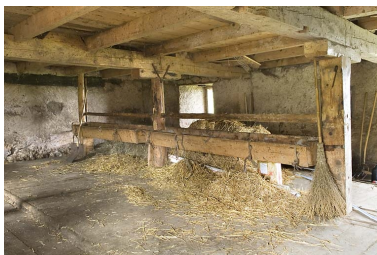
Etable. Phot. Jérôme Mongreville IVR43_20082500939NUC2A
