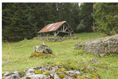
"Couvert" de la Cafaude. Phot. Jérôme Mongreville IVR43_20082500952NUC2A
