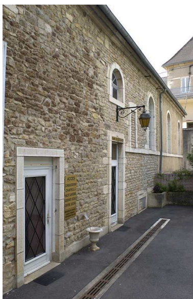
Façade postérieure. Phot. Michel Thierry IVR26_20032100407NUC2A
