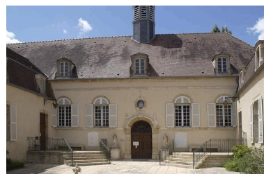
Corps central de la façade principale. Phot. Michel Thierry IVR26_20032100403NUC2A
