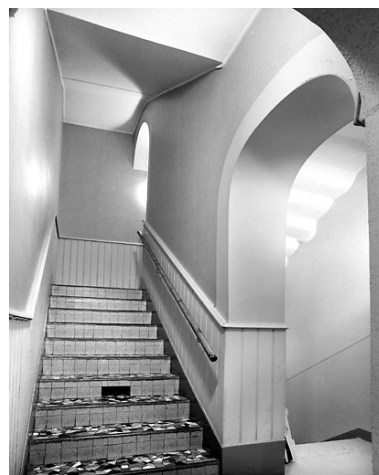
Escalier. Phot. Yves Sancey IVR43_20033900757X
