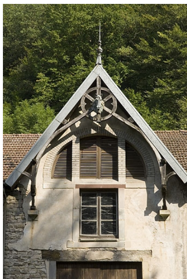
Ecuries. Pignon central. Phot. Jérôme Mongreville IVR43_20067000737NUCA
