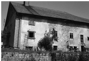
Façade postérieure. Phot. Gilbert Poinot IVR43_19752501021Z
