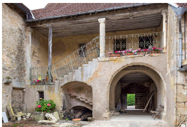
Façade postérieure. Phot. Sonia Dourlot IVR43_20157000328NUC2A
