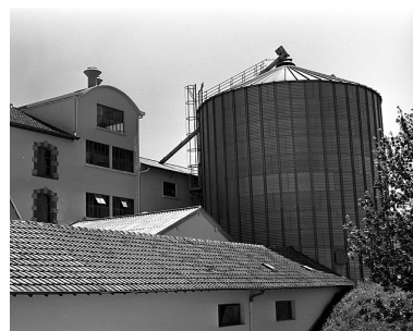
Silos. Phot. Jérôme Mongreville IVR43_19963900434X
