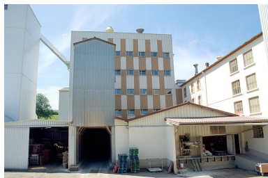
Magasins industriels. Phot. Jérôme Mongreville IVR43_19963900424ZA
