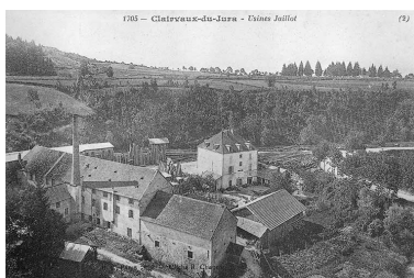
Clairvaux-du-Jura - Usines Jaillot. Phot. Jérôme Mongreville IVR43_19963900003X
