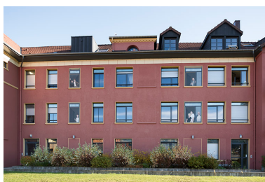
Façade antérieure. Phot. Sonia Dourlot IVR43_20172501829NUC4A
