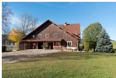
Façade antérieure (sud). Phot. Sonia Dourlot IVR43_20172501656NUC4A
