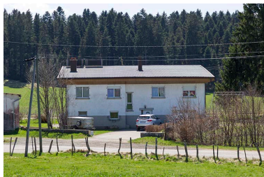
Façade antérieure. Phot. Sonia Dourlot IVR43_20152500951NUC2A
