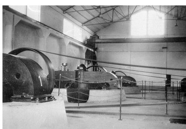
Station. Turbines. Phot. Yves Sancey IVR43_19883900588Z
