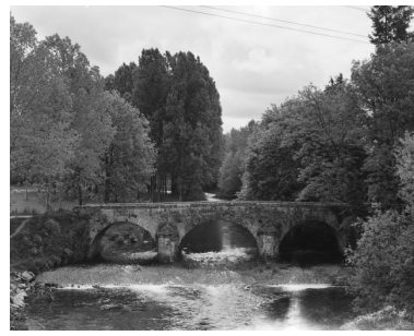
Face aval, vue de face. Phot. Yves Sancey IVR43_19813900072X
