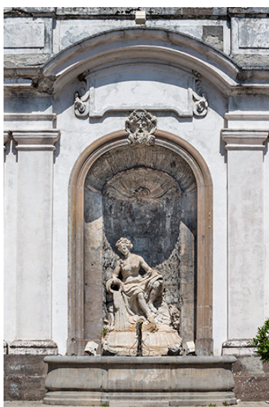
Niche centrale. Phot. Jérôme Mongreville IVR43_20223900454NUC4A
