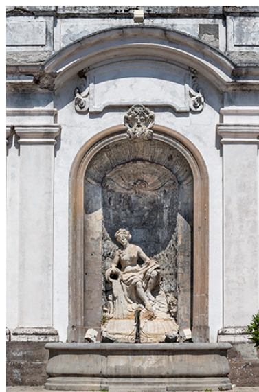
Niche centrale. Phot. Jérôme Mongreville IVR43_20223900454NUC4A
