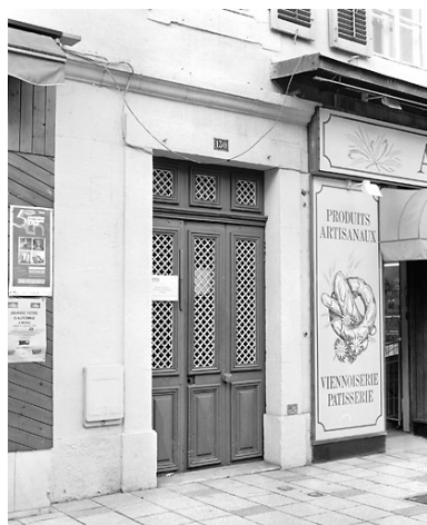
Porte principale. Phot. Yves Sancey IVR43_20033900780X
