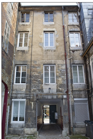
Logis principal : façade postérieure. Phot. Yves Sancey IVR43_20102500459NUC2A
