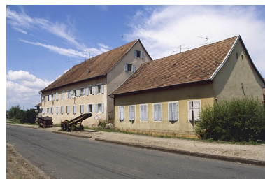
Façades sud. Phot. Yves Sancey IVR43_20019000357ZA
