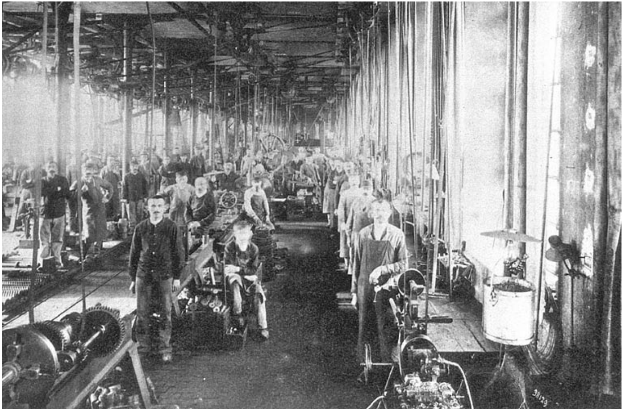
Atelier de construction.
