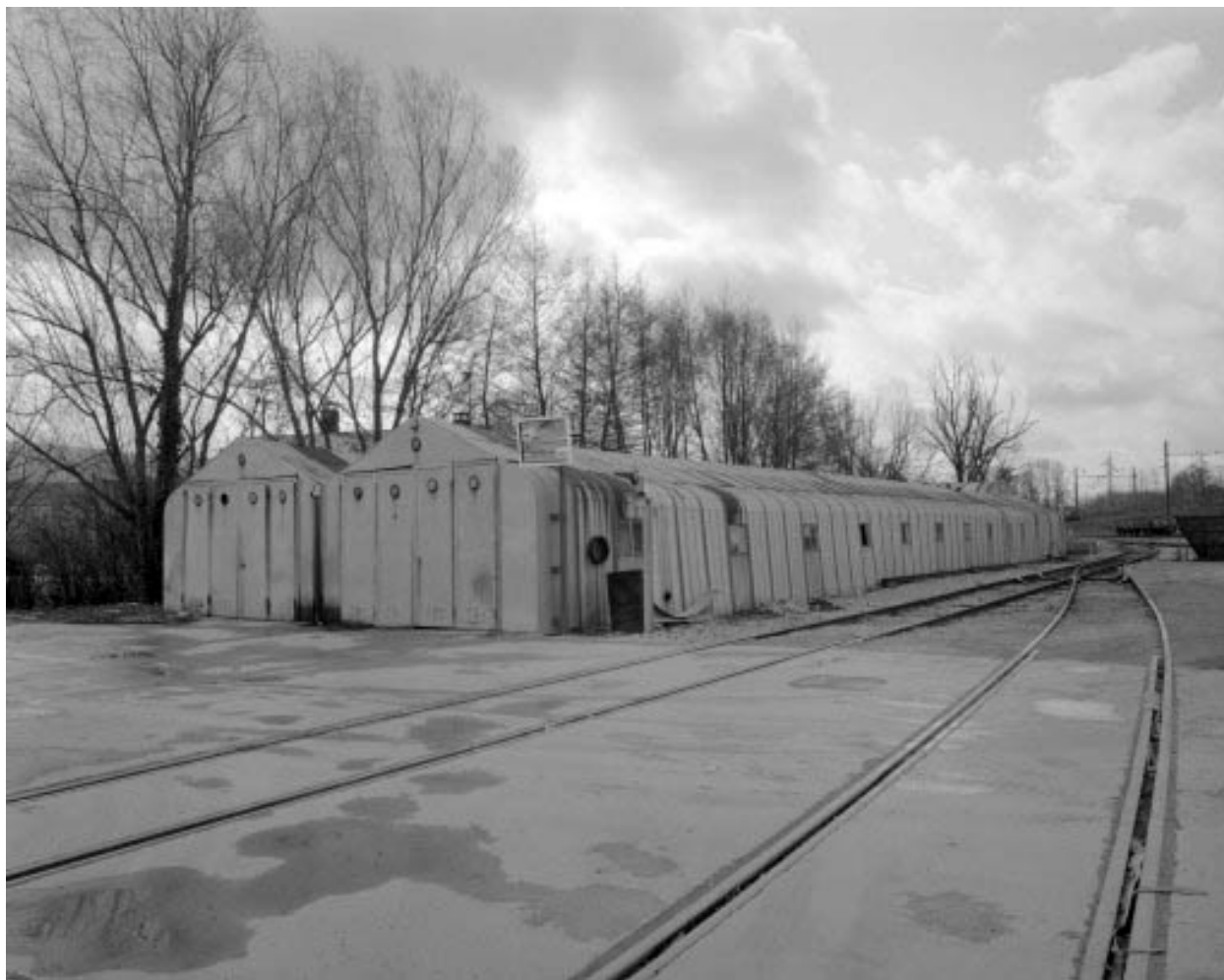
Baraques de chantier (F).
