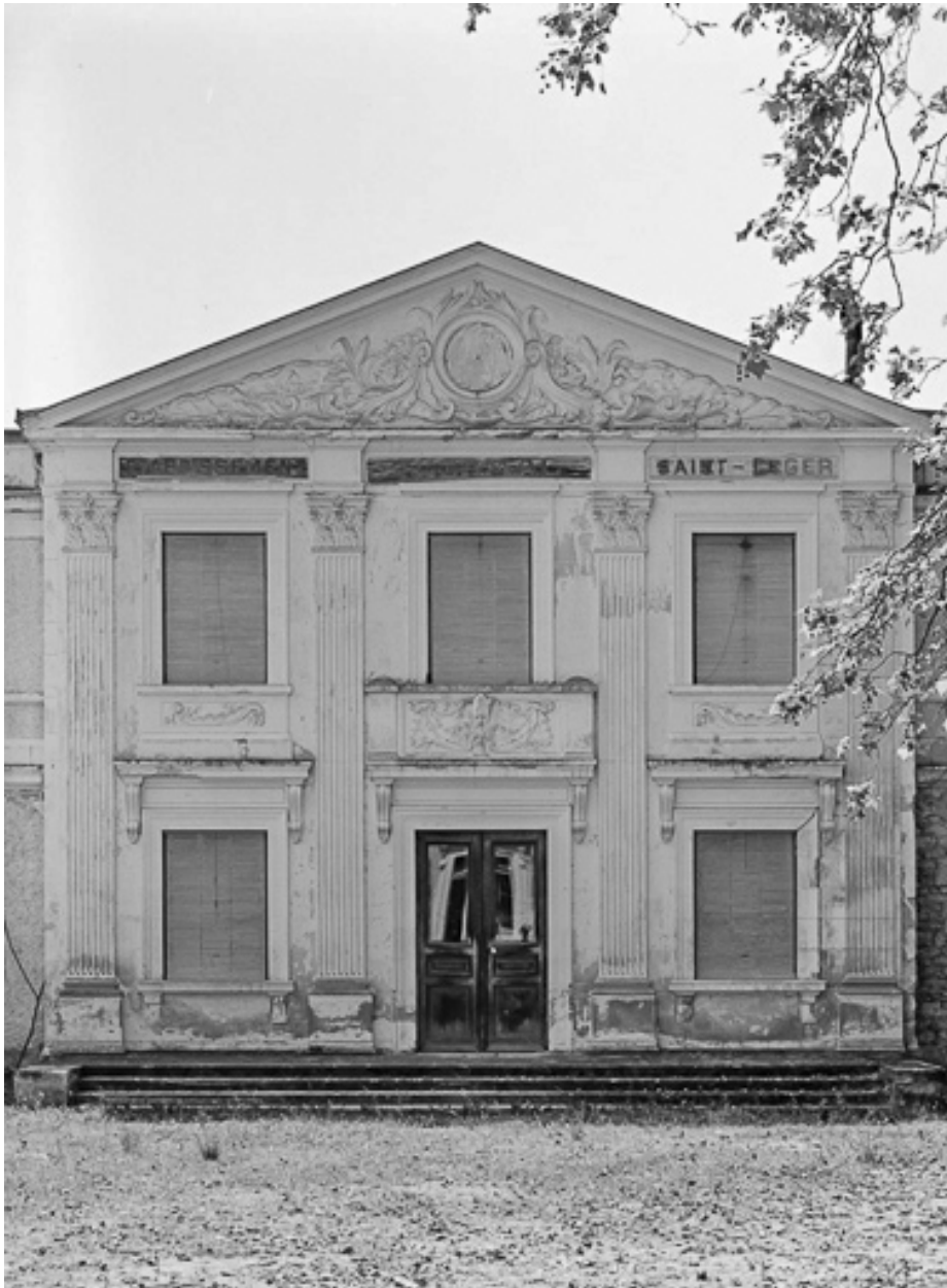
Façade antérieure, avant-corps.
