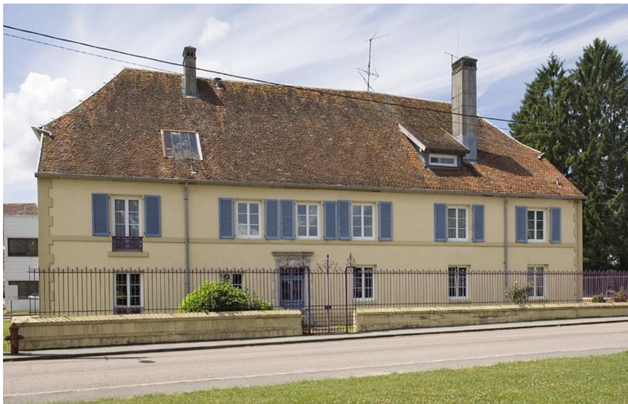
Logement patronal. Façade est.
