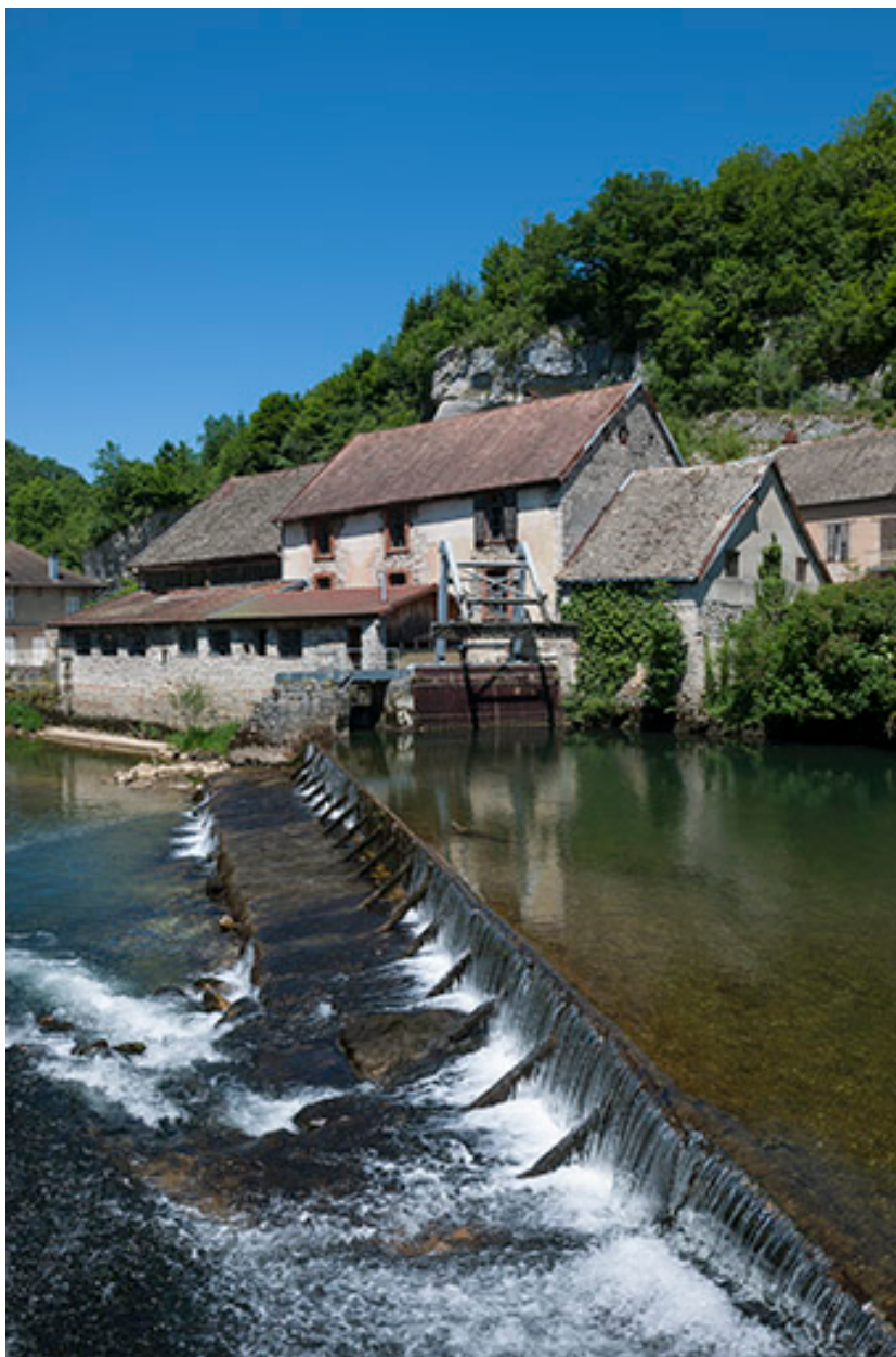
Atelier Auguste Louvrier, Lods.
