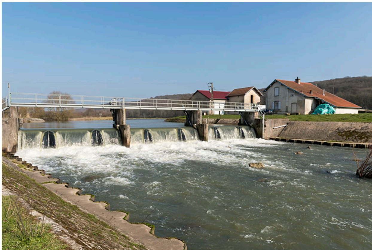
Barrage mobile, Cendrecourt.
