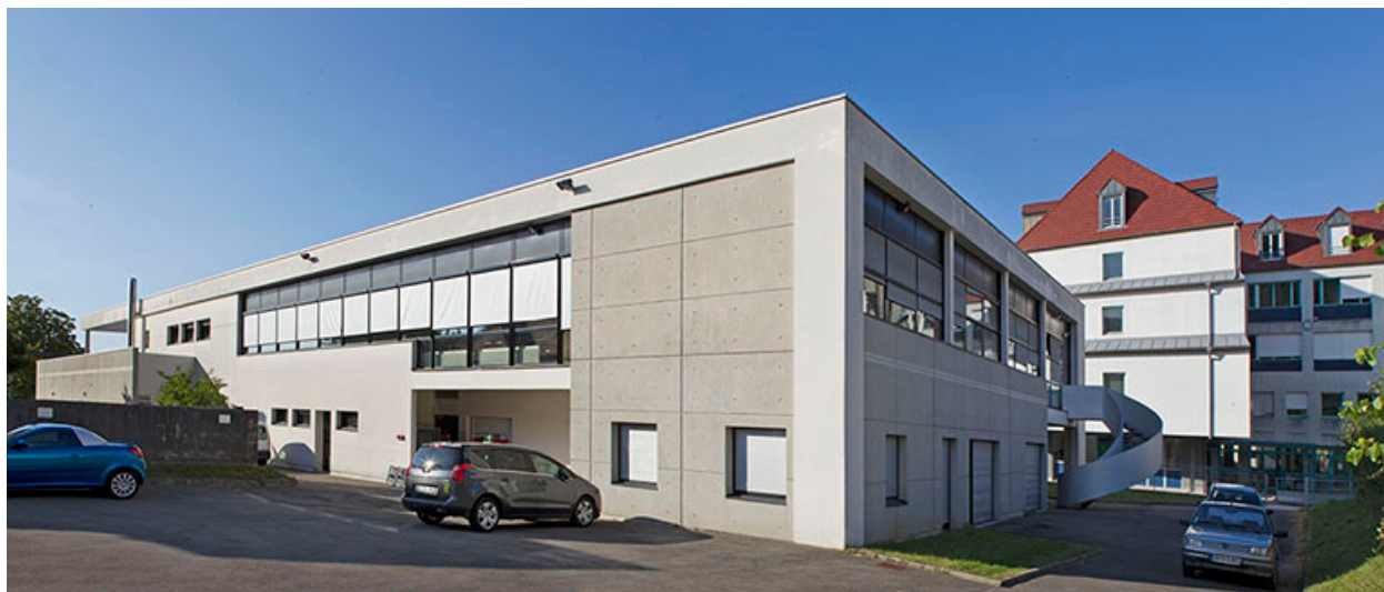
Restauration : façade Est.
