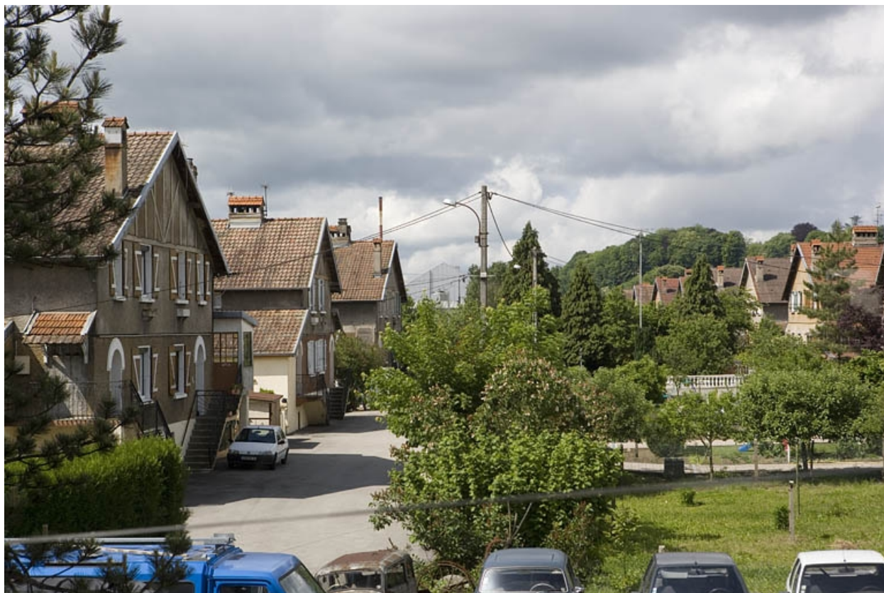
Cité Lehmann. Place de Chemontey.
