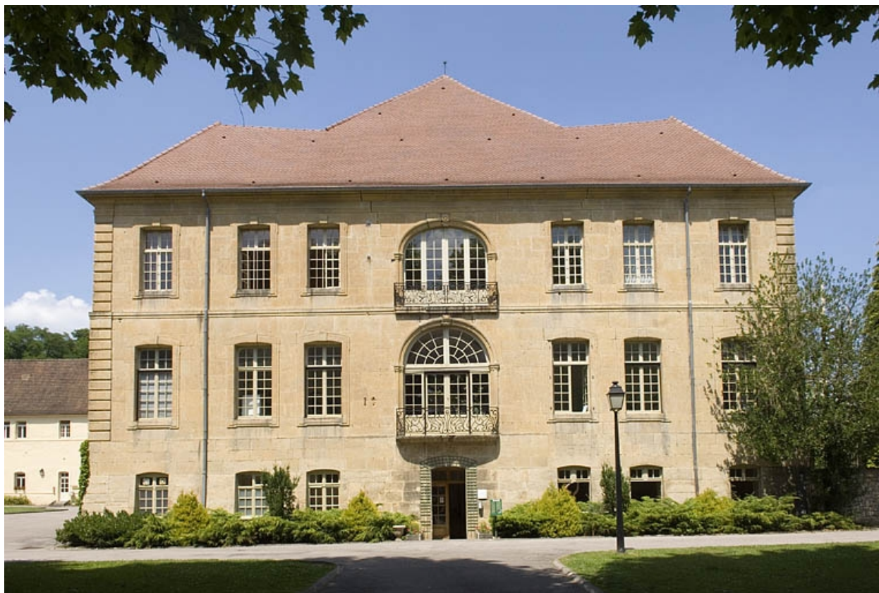
Logis abbatial. Façade sud.
