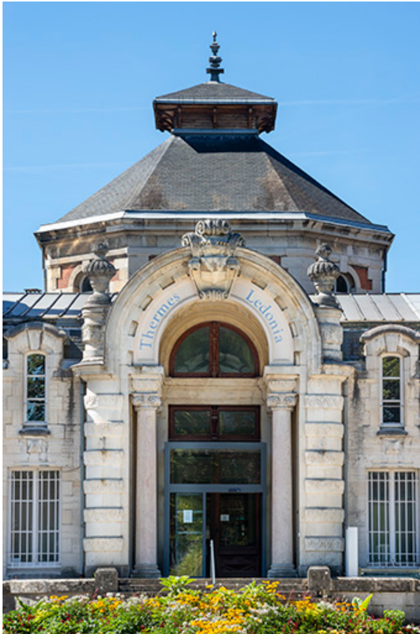
Façade principale, portail.
