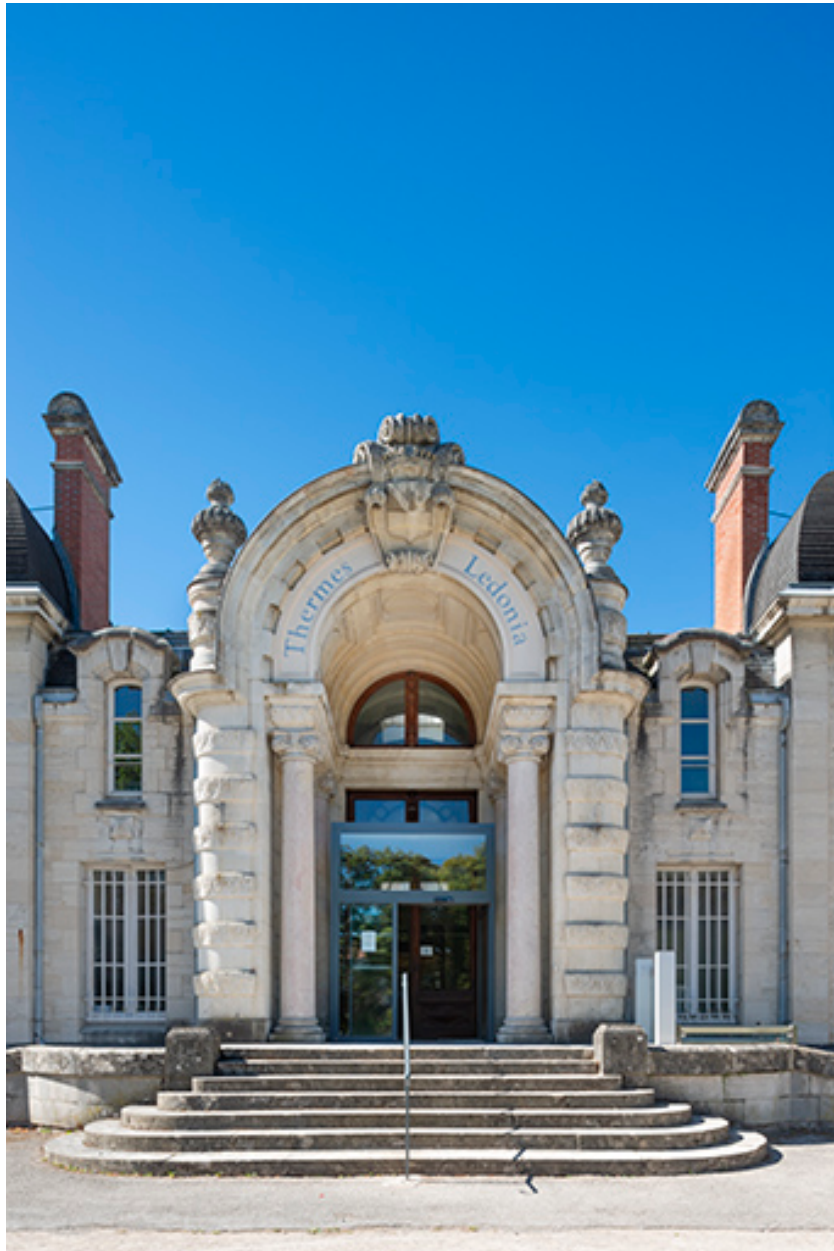
Façade principale, portail.
