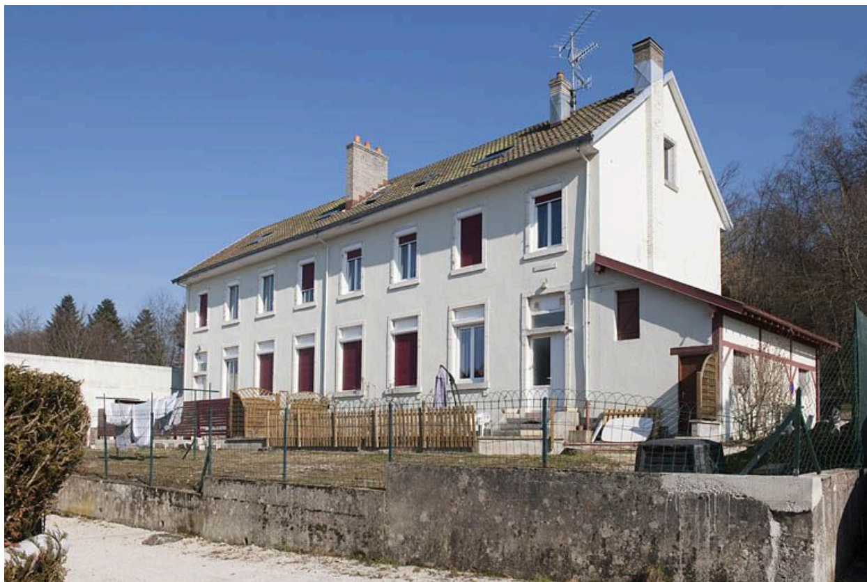
Ecole. Façade ouest.
