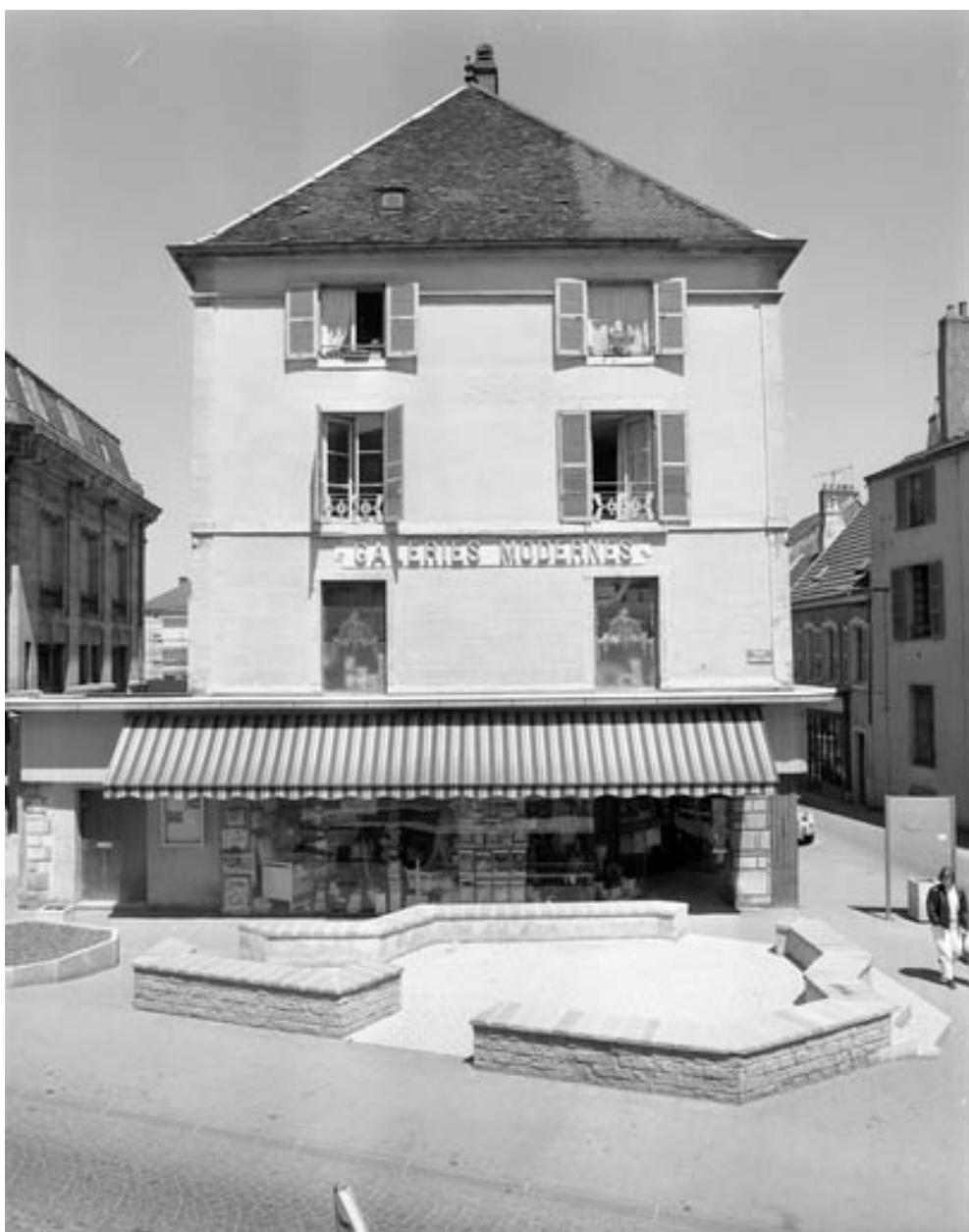
Façade principale, de face.
